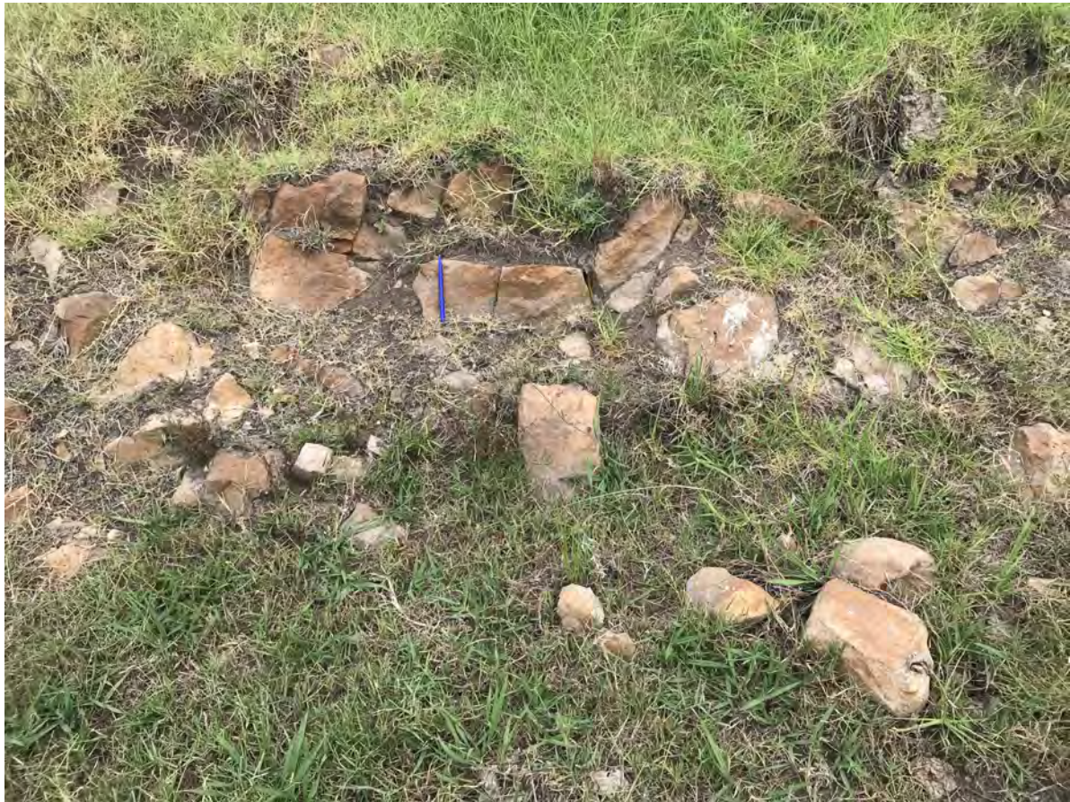
Photo 5 - Latite/residual soil exposed in dam wall
